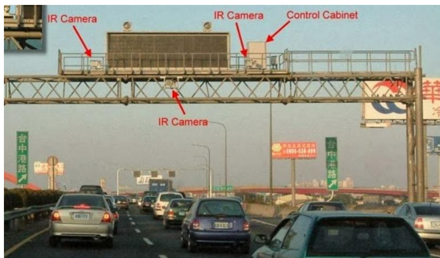
Try to install the cameras perpendicular to the street and expect to capture plates
